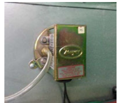
Differential Pressure Switch
