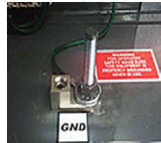
Main Load Block (top) and Ground Block
